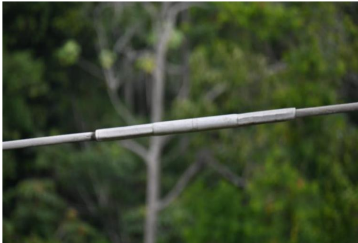
Figure 6. Inspection of splices in conductor cables [2].
