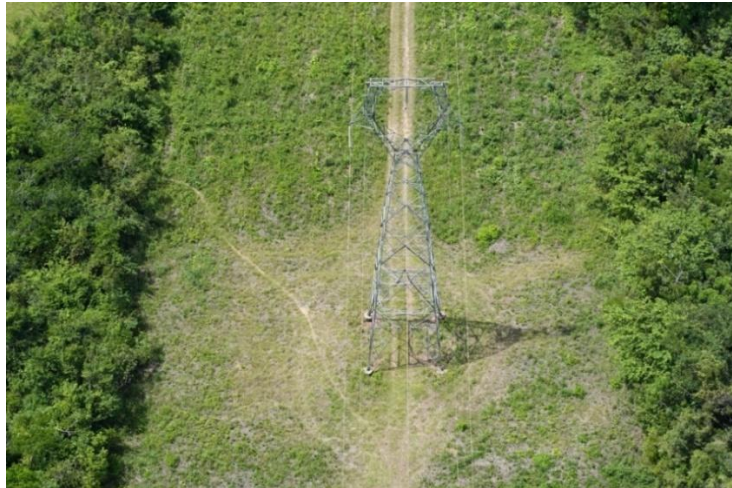
Figure 5. Digital photography of aerial inspection [2].
